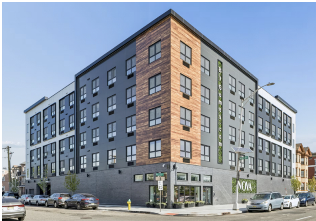
Nova by Gomes at 1213-1221 Mayor Kenneth A. Gibson Boulevard. Developed by Gomes Group.
